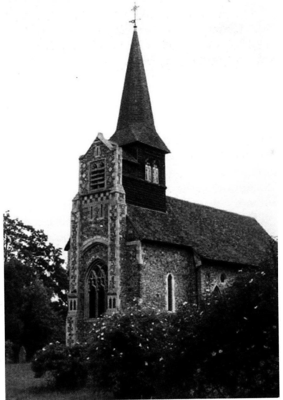
Fig. 14 All Saints, Great Braxted, Essex: west tower partially rebuilt by the Revd Ernest Geldart, 1883-4.
